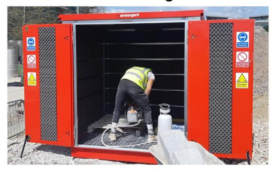
PORTABLE SOLUTION TO PROVIDE A SAFER SCENARIO FOR THOSE CUTTING MASONRY BASED ITEMS SUCH AS PAVING SLABS, CURBSTONES AND TILES, AS WELL AS THOSE AROUND IT.
