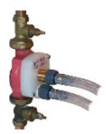
2c. Across the "tails" of a radiator (having drained and disconnected the radiator) using appropriate 1/2" or 3/4" BSP adaptors to connect to the valves. The radiator valves should be closed to isolate the flushing pump from the system until
