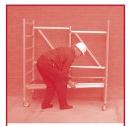
4. Locate the trap platform onto the lowest rungs of the two end frames. Ensure unit is level by placing on level ground or is leveled using adj legs (if fitted) and a spirit level.
