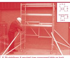
8. Fit stabilisers if required (see component table on back page) to each corner of the tower to increase the effective base dimension "A" & "B". They must be fitted so that when viewed from above the largest square is formed. Ensure that the wing nuts are tight so that it is not possible to move the stabilisers without slackening the wing nuts. Do not over tighten them as this may distort the tube.
