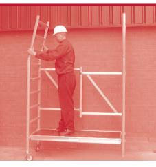
6. If required fit a second extension frame in the opposite end frame engaging the conical fittings in the same manner
