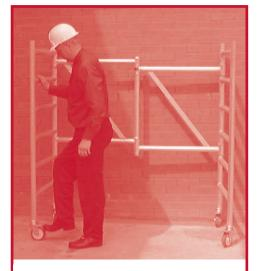
$\ensuremath{\mathsf{3.Apply}}$  the brakes by pressing the brake bar downwards
