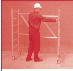
2. Stand the unit upright and push the two end frames apart so that the hinged bracing member is fully extended and the frame forms three sides of a rectangle when viewed from above. The locating holes at the top of the frames should be facing inwards.
