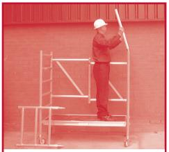
5. If required (see component table on back page) add an extension frame by locating the conical fittings of the extension frame into the top of the end frame of the folding unit ensuring that the pegs engage in the holes provided.
